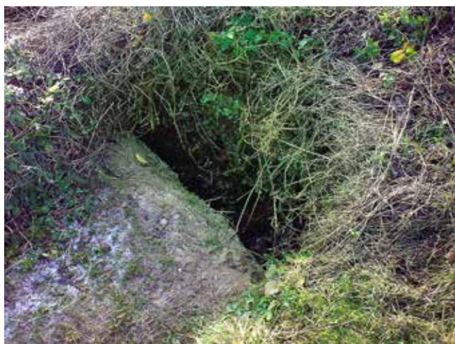
Until recently the entrance at the top of the stairs was the only way in to the shelter
